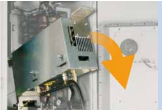
4. Modules can be popped out towards the front.
